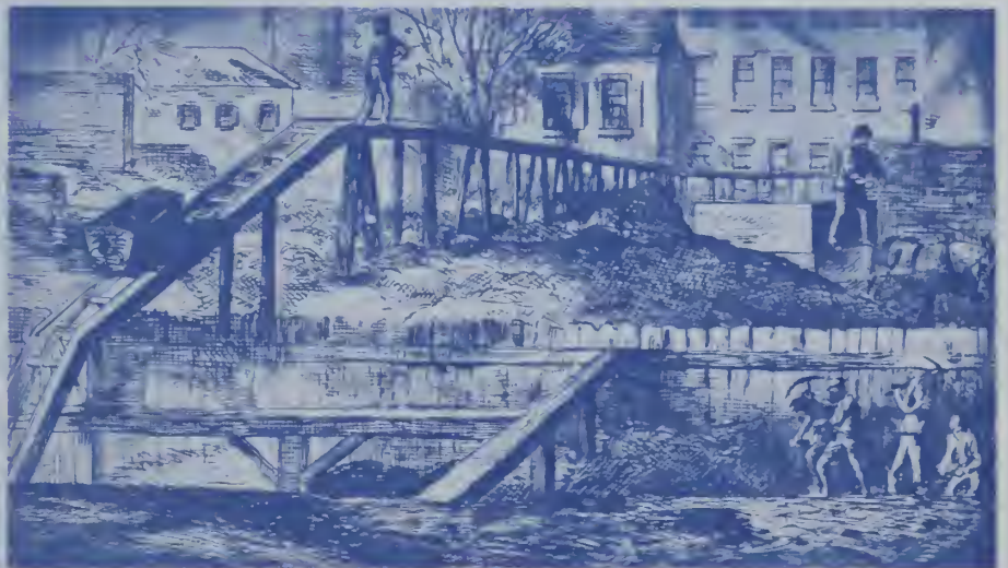
This old print from "The Daily Graphic" of May 2, 1873, shows the method of removing material from the site of the Brooklyn anchorage.
